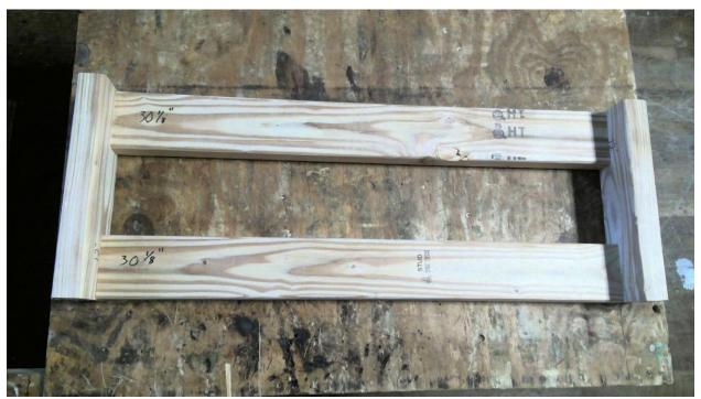
It's helpful to drill pilot holes to keep the short boards from splitting. Place two screws through each side of each small board into the end of the longs boards forming the brace pictured above
